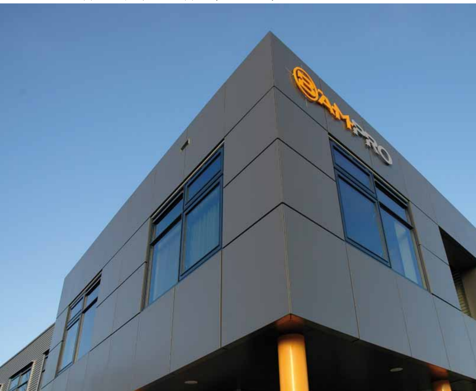
Bam, Hardinxveld (NL) | Architect: Jan Buijs, Hardinxveld (NL) | Limeparts: aluminium powder coated
